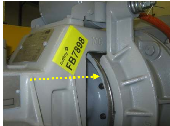
Photograph 4. Level 32: Plant room, Rocker covers to original Chiller unit No.3; Compressor 1 - Oil gaskets (Refer to sample CA3121 - NAD).
