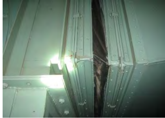
Photograph 10. Level 31 - Hydraulics riser; Gasket to drain/stormwater pipe: Non-asbestos gasket. Refer to sample CA3122 - NAD
