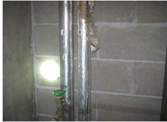
Photograph 12. Levels 17 to 33: Building core; C.W and H.W Service risers; Vertical Condenser and Hot Water pipes - SMF insulation to pipes (foil lined)
