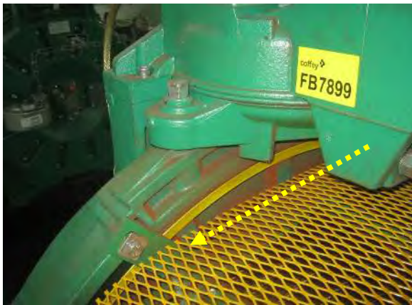
Photograph 5. Level 32 Plant room; Chiller pipe network – Flow and return pipe connections; Vulcanised gaskets to flange pipe junctions and shut-off valves.
