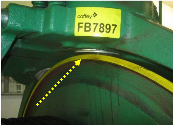
Photograph 3. Level 33: Lift Motor room; Lift Motor L.M No.8 ('KONE') - Brake callipers; Brake compound linings. (Refer to sample FB7899 - NAD).
